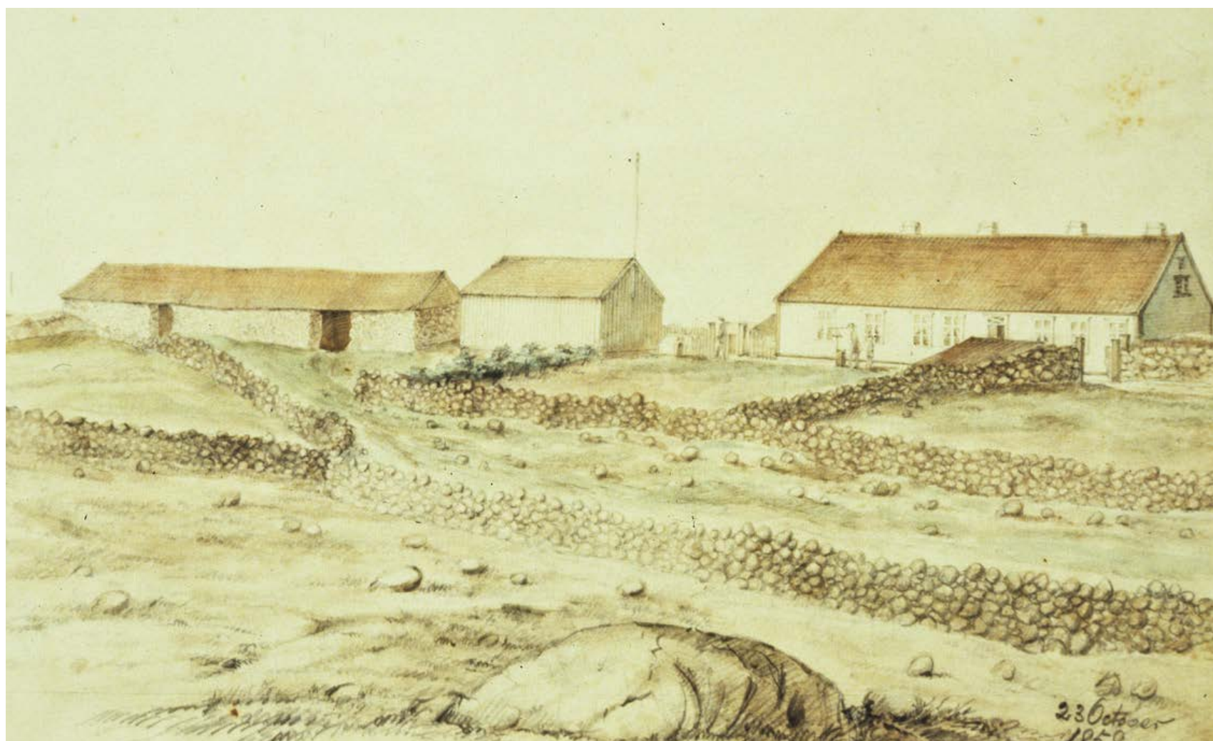
Fig. 3. The Old Parsonage in 1858. The main house was built up again in 1790 after a fire. The building signals high status, with its white-painted walls, red roof tiles and large glass windows. Note the high drystone fences – perhaps originating from the now lost cairns recorded in 1842 by Kraft? Water colour by Gabriel Monsen. (Photo courtesy of Stavanger Museum.)
