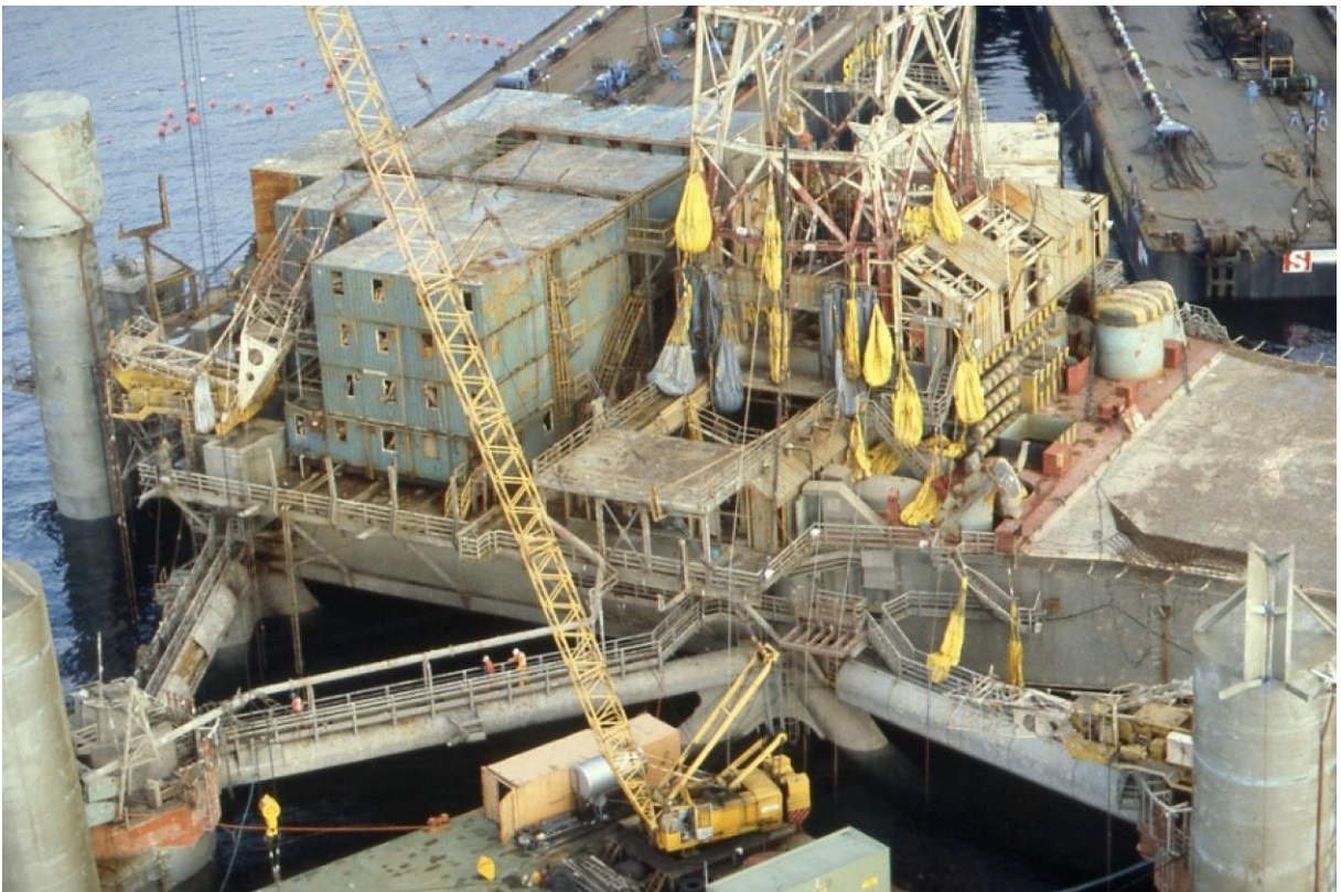
Photo 9. Parts of the platform deck. Photo: Stavanger A. V. Institutt as.
