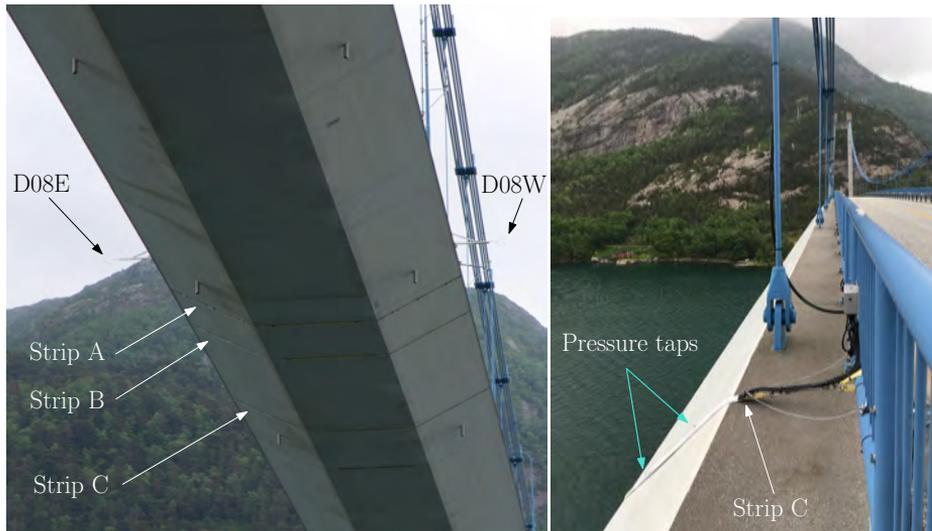
Figure 3.15: The pressure strips as seen from the base of the North tower (left panel) and a side view of one end of the strap and corresponding anchoring elements, showing also two tapping points (right panel). Photos by J.T. Snæbjörnsson - UiS.
