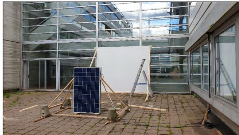
Figure 3. The panel cladding installation phase.
