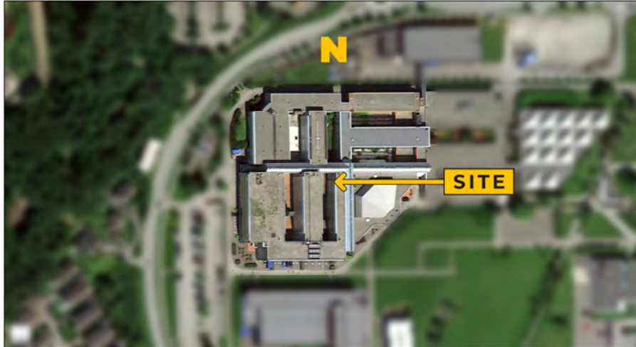
Figure 3-2 A picture of the site and the system
