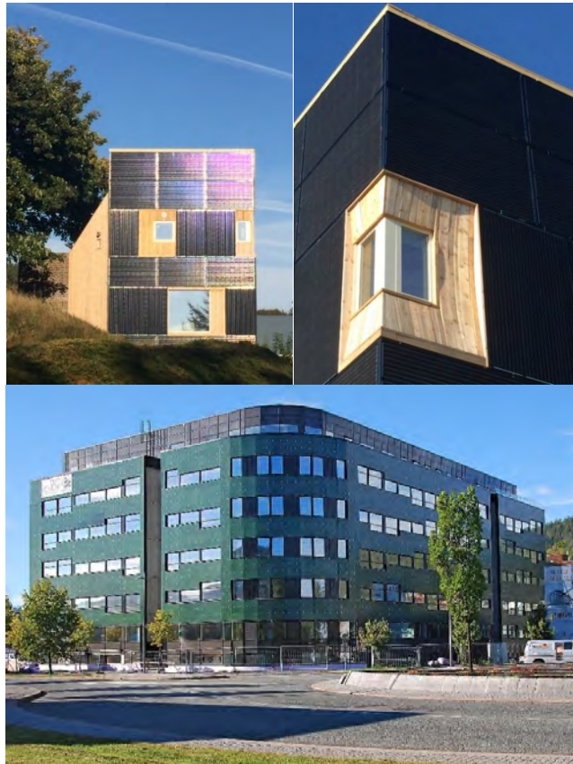
Figure 1-2 Examples of building equipped with BIPV systems [13, 14]
